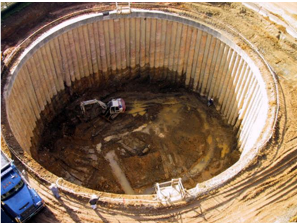
Graphic 3-7 Secant piled tunnel shaft construction
