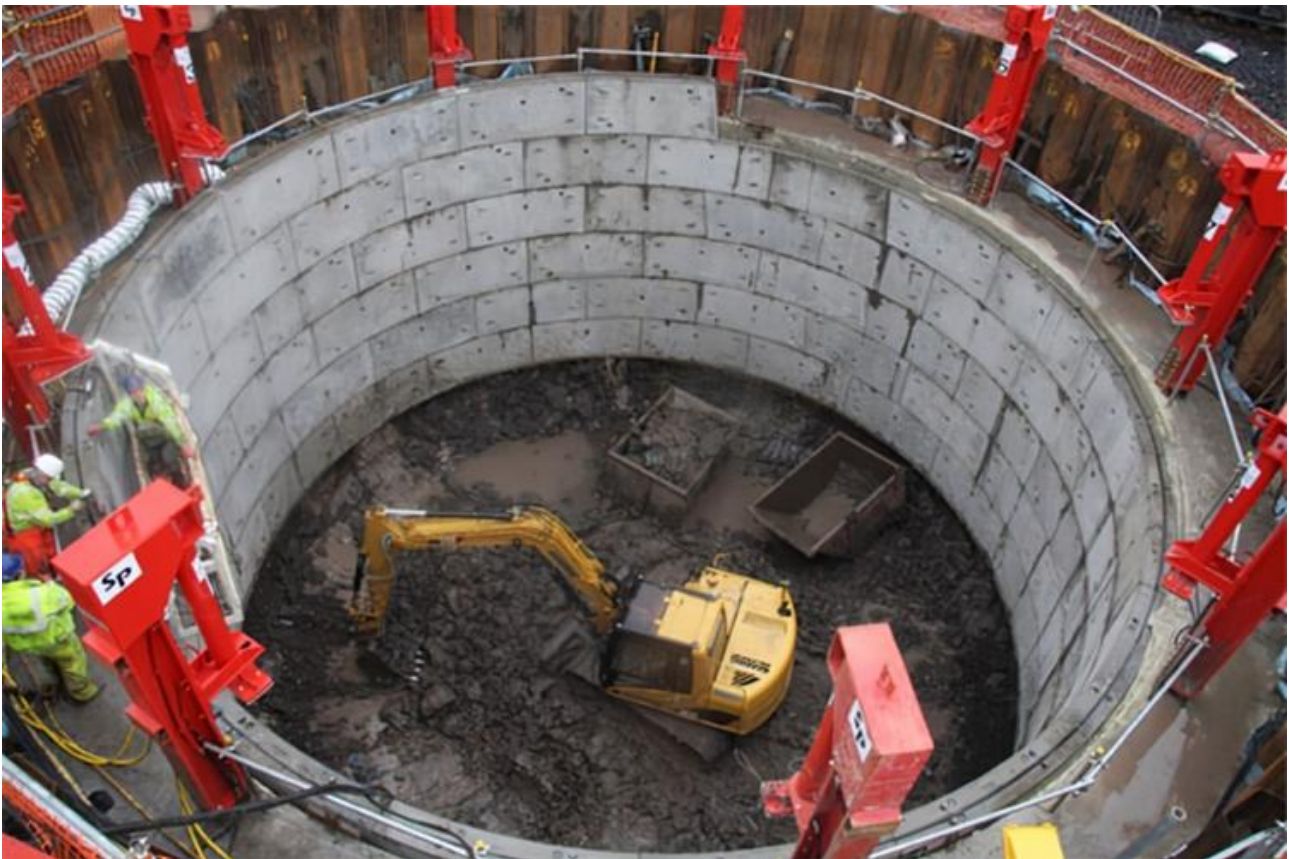
Graphic 3-5 Open caisson sinking tunnel shaft construction
