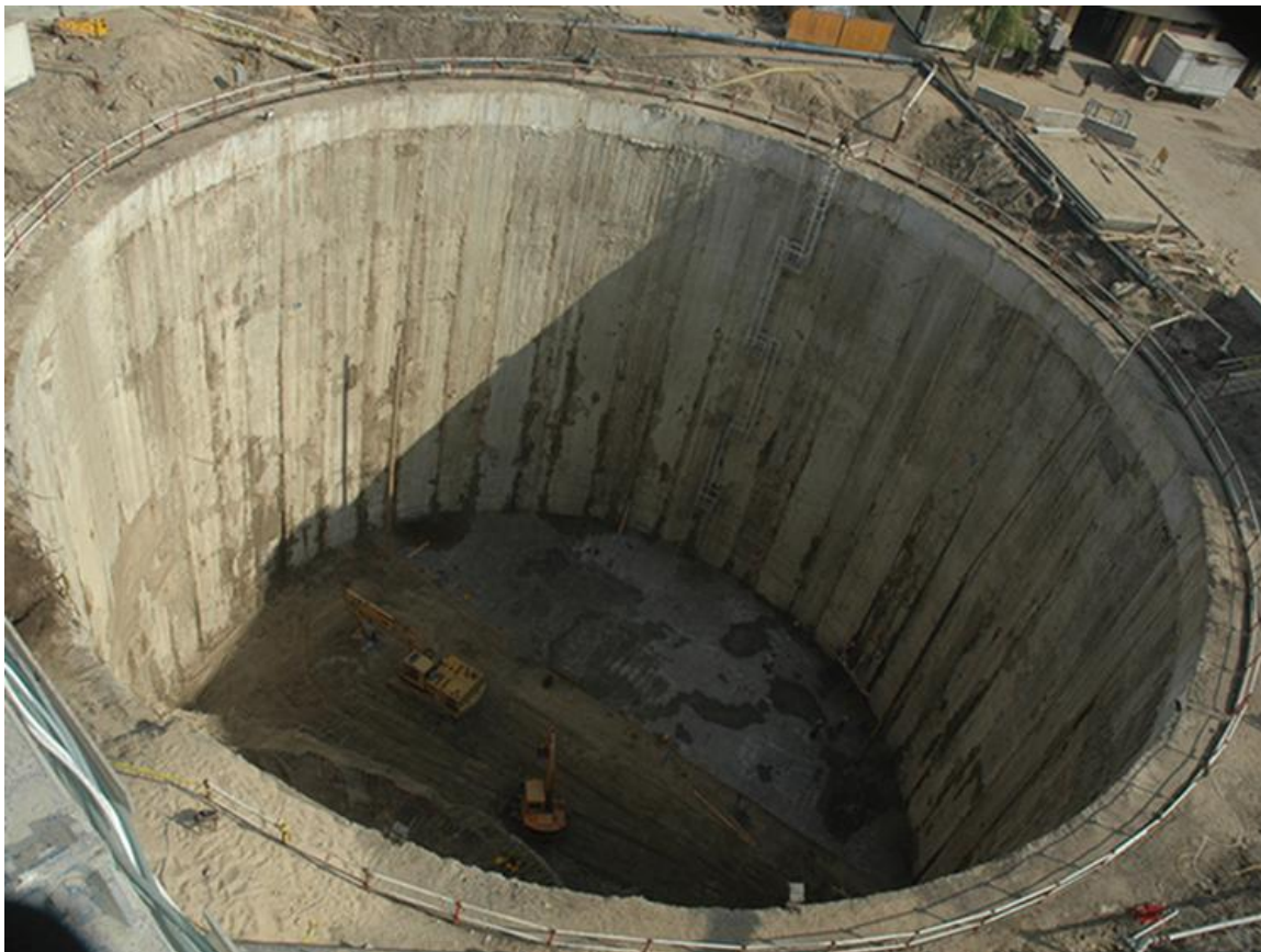
Graphic 3-8 Diaphragm tunnel shaft construction
