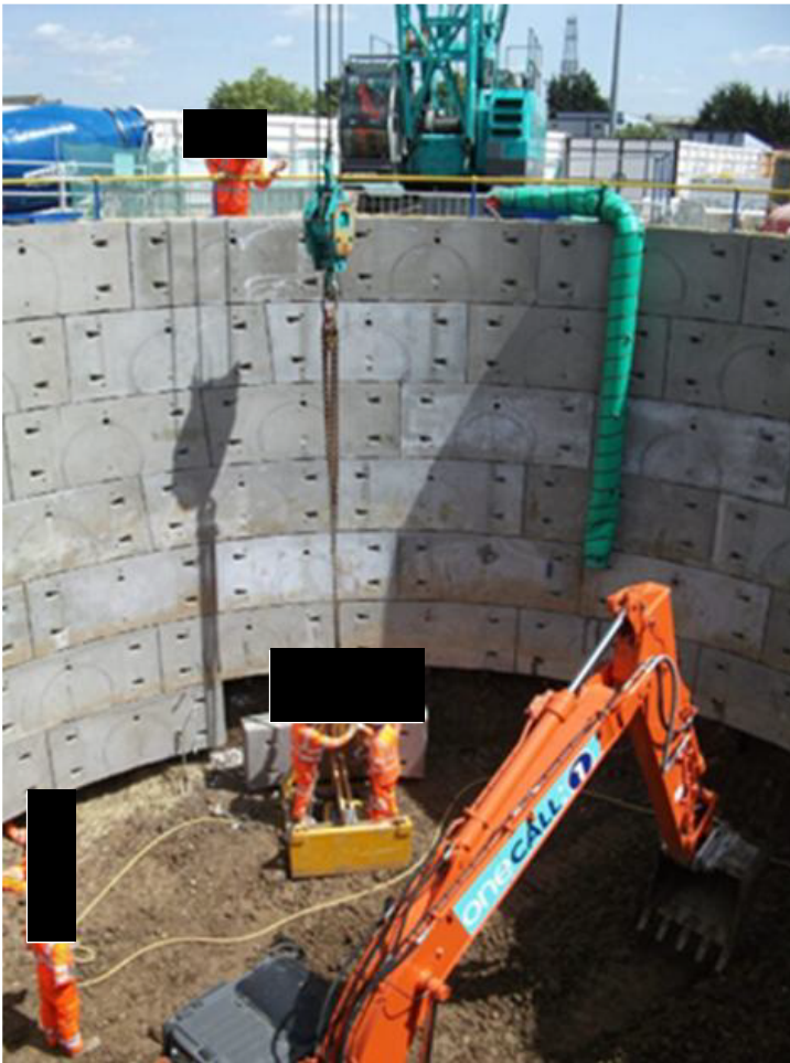
Graphic 3-6 Underpinning tunnel shaft construction
